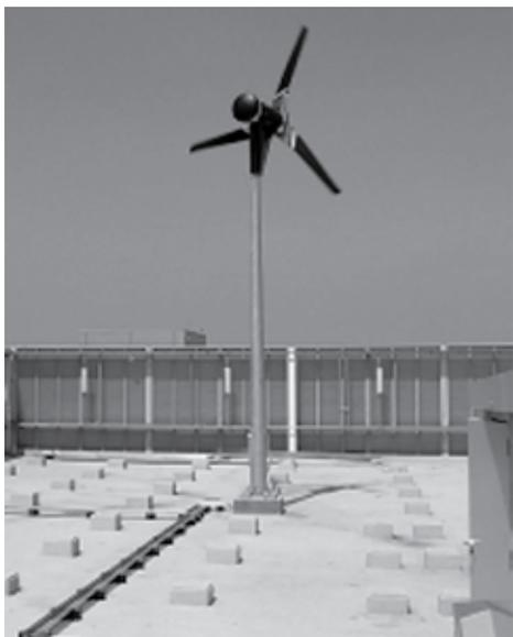
The integration of solar photovoltaics and a wind turbine into the plant deck on the top floor of the Croydon Centrale shopping centre.
